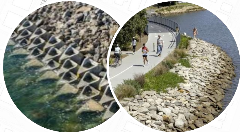
Ecological rock revetments
