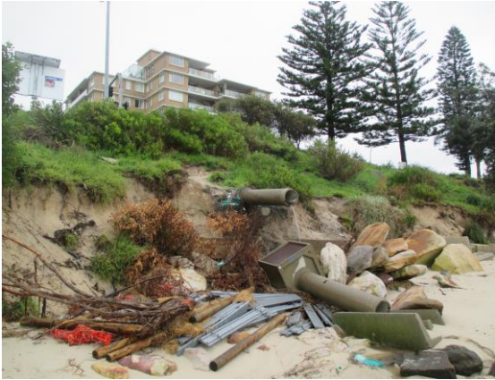
Figure 1.3: Heavily eroded shoreline, foredune scarping and ad-hoc rock at President Avenue
