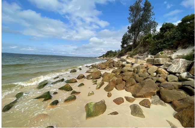
Figure 1.3: Heavily eroded shoreline, foredune scarping and ad-hoc rock at President Avenue
