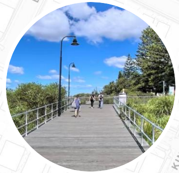
1. Boardwalk terminates abruptly
