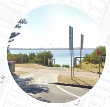
2. Vehicular access to eroding beach
