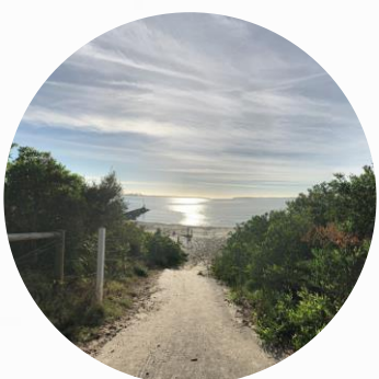
7. Pedestrian access to beach (non-DDA compliant)
