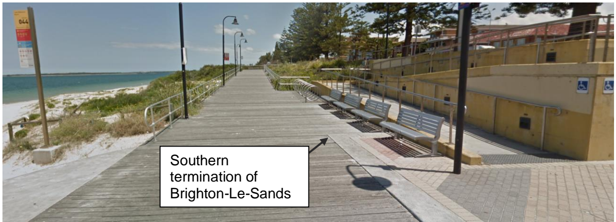
Figure 5.1: Southern termination of Brighton-Le-Sands seawall
