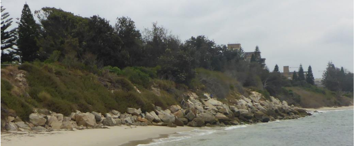
Figure 5.3: Banks St rock works in 2019.
