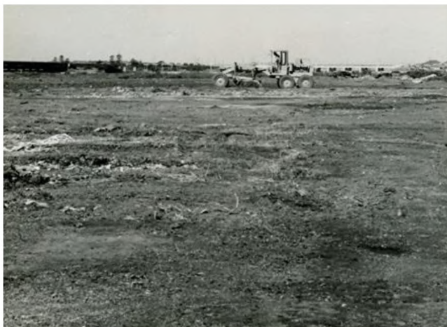
Figure 10 - Photo taken during development of park, after completion of garbage filling, levelling of land near the sewer carrier. September 1959 (Source: Bayside Library)
