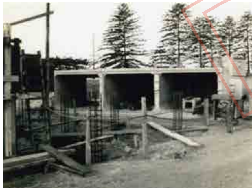
Figure 8 - Work underway on the building of the triple sewer at Kyeemagh after the reclamation and diversion of the Cooks River, late 1940s (Source: Bayside Library)
